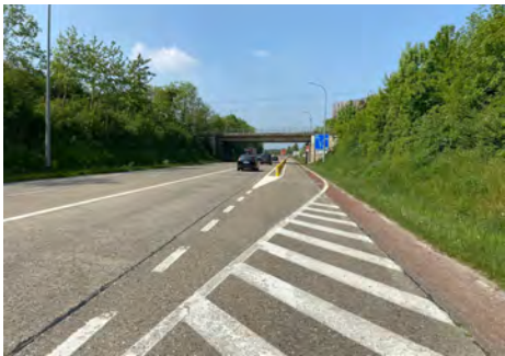
Exit towards entrance N3 Haspengouwlaan
